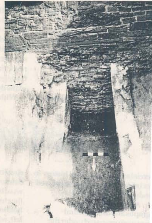
Stone foundations of the 1835 entrance way at Benares. Note the blocked doorway. (Photo: Dena Doroszenko)
