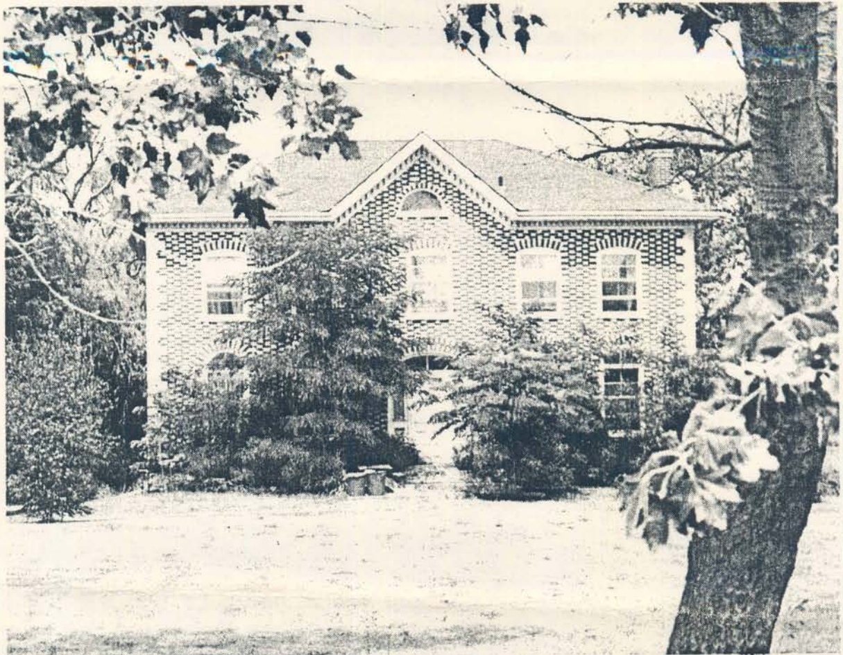
The German style of brick-laying used in Sunnyside Cottage is uncommon in Canada.
