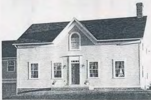
At a glance you might think the Smiths' home was built in the 1830s, but in fact it's just over a year old. It takes its inspiration from an early house, and many of the structural and trim components are recycled.
