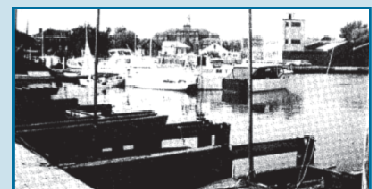
Cribwork of the old ferry slip serves as the marina in the 1960s/70s.
