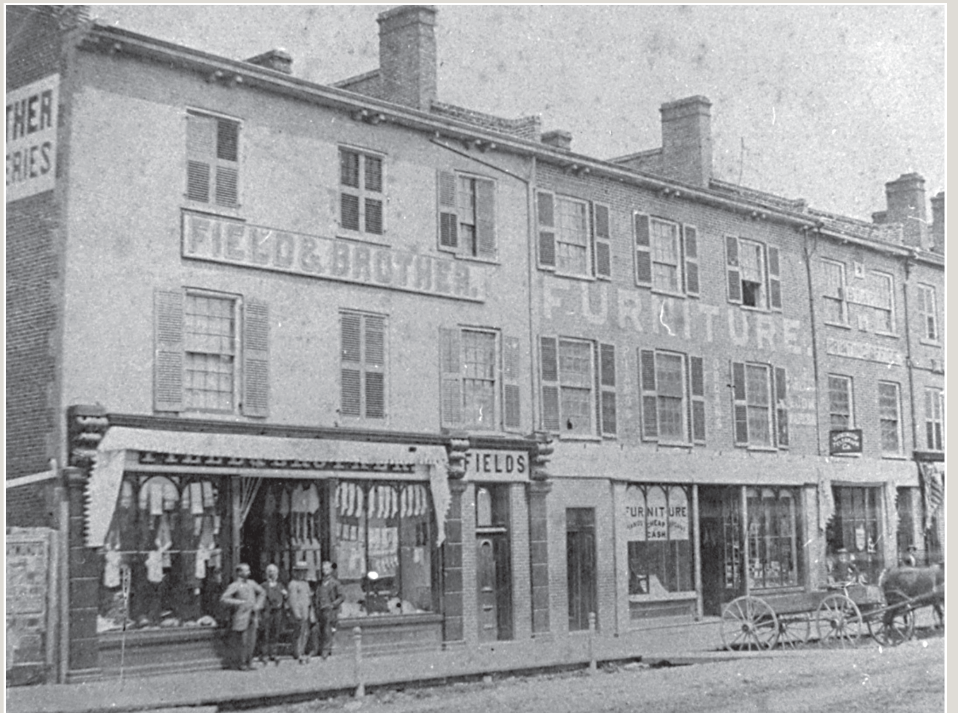
Field and Brother's storefront on north side of King Street opposite Victoria Hall
