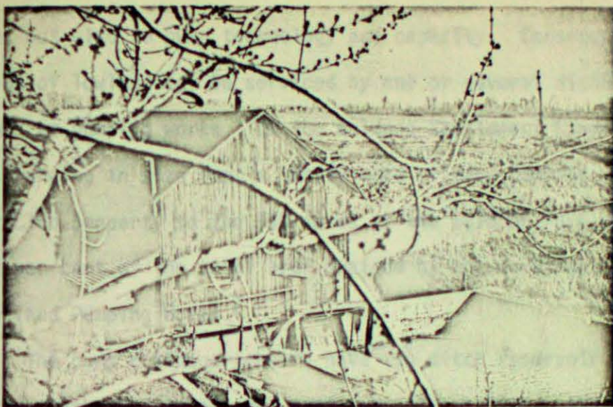
Figure IV-3. ROSE PUMP-HOUSE; GRAVITY DRAINAGE GATE AT LOWER CENTRE; TAIL-RACE OUTLET TO LITTLE BEAR CREEK IN THE FOREGROUND (Source: see Appendix A).
