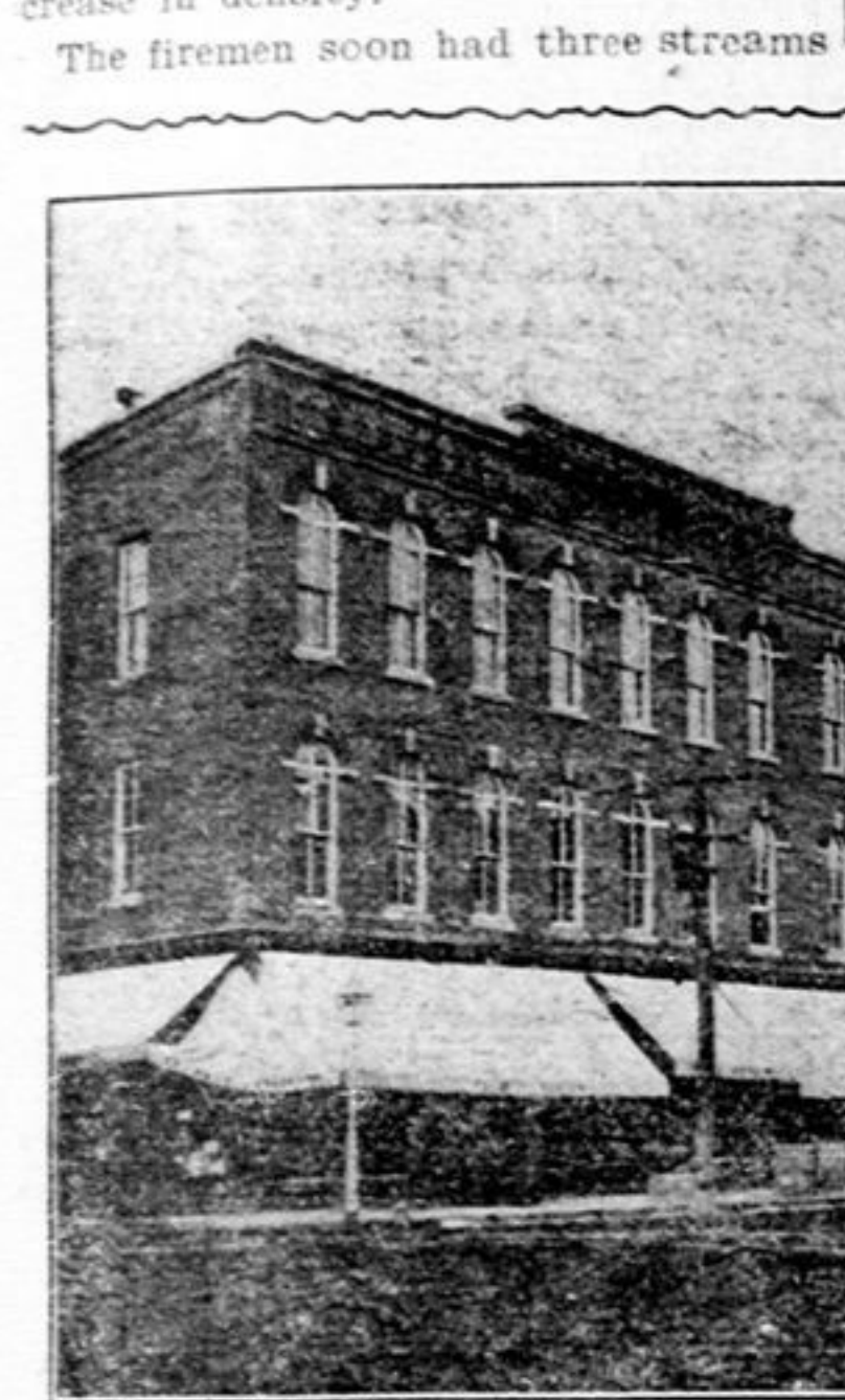
SCENE OF TO-DAY'S DESTRUCTIVE FIRE
