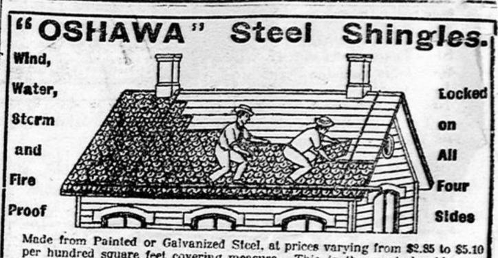
per hundred square feet covering measure. This is the most durable covering on the market, and is an ideal covering for Houses, Barns, Stores, Elevators, Churches, etc. Any handy man can lay the "OSHAWA" shingles. A hammer and snips are the only tools required.
