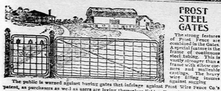
STEEL GATES The strong features of Frost Fence are combined in the Gates. A special feature is the frame of continuous steel tubing. This is rame with elbow corners and malleable castings. The heavy wire filling insures
