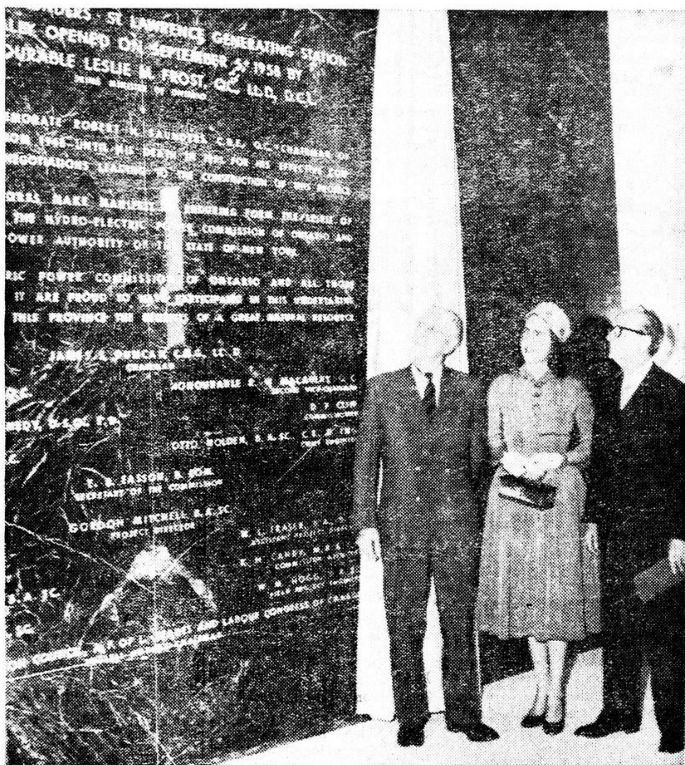
(OTT 2) CORNWALL, ONT., SEPT. 5 — UNVEILING — The St. Lawrence Power Project was officially opened in Cornwall, Ont., today. The project has adjoining powerhouses — the Robert H. Saunders - St. Lawrence Generating Station, on the Canadian side, and the Robert Moses Power Dam, on the American side. Left to right in this picture are: Premier Leslie Frost of Ontario; Mrs. Robert Falconer, daughter of the late Mr. Saunders, Chairman of the Hydro-Electric Power Commission of Ontario from 1948 until his death in 1955; and James S. Duncan, present Chairman of the Commission.
