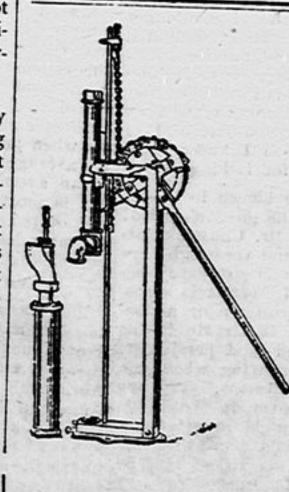
Buck's Patent Ec-Chain Lift centric Pump.
