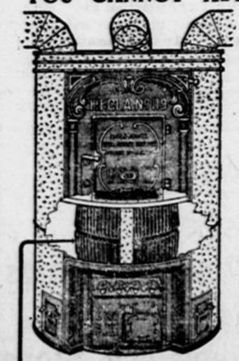
The "Hecla" will do this: It is built to save coal at every point, but the big coal-saving feature is the Steel Ribbed Fire Pot. By adding Steel Ribs to the Fire Pot the surface which radiates heat is increased three times.
