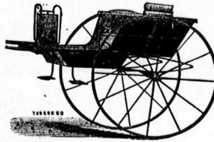
TWO SIZES, SURREY AND PHAETON BODIES The Shafts are attached to body by the Perry Compensating Spring. The result of the action of these Springs is no horse-motion in the cart, and no cart-
