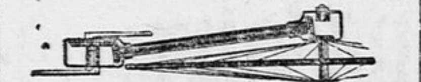
GEAR FOR CHAINLESS BICYCLES.
