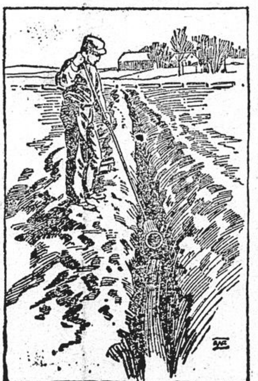
FIG. 2.—GOOD WAY TO LAY TILE.
