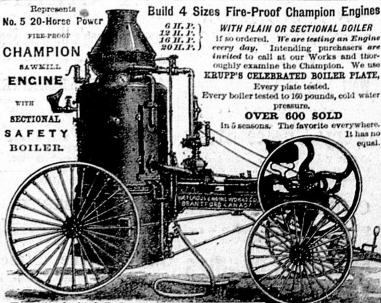
The sectional safety boiler is manufactured expressly for the "North West" trade. This boiler is so arranged that it is readily taken apart in sections enabling purchasers to clean thoroughly every part of it and prevent burning out. We know from experience this is absolutely necessary with the alkaline waters of the great Western prairies. Largely used by the Pacific Railway Company and all the large Colo-
