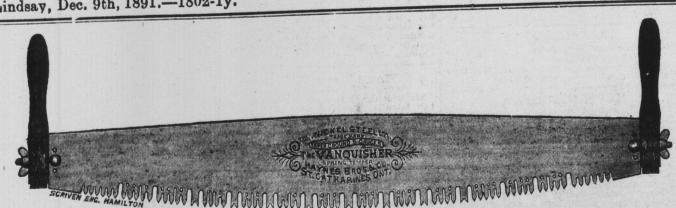
These Saws are made from the best Nickle Steel Spring, tempered; fully warranted; require no set. We also keep in stock a full line of SHELF HARDWARE, and everything in the BUILDING LINE.
