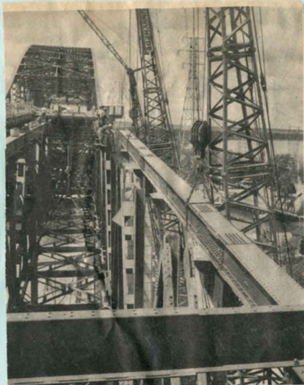
Aldershot Equipment worked on Skyway Bridge.
