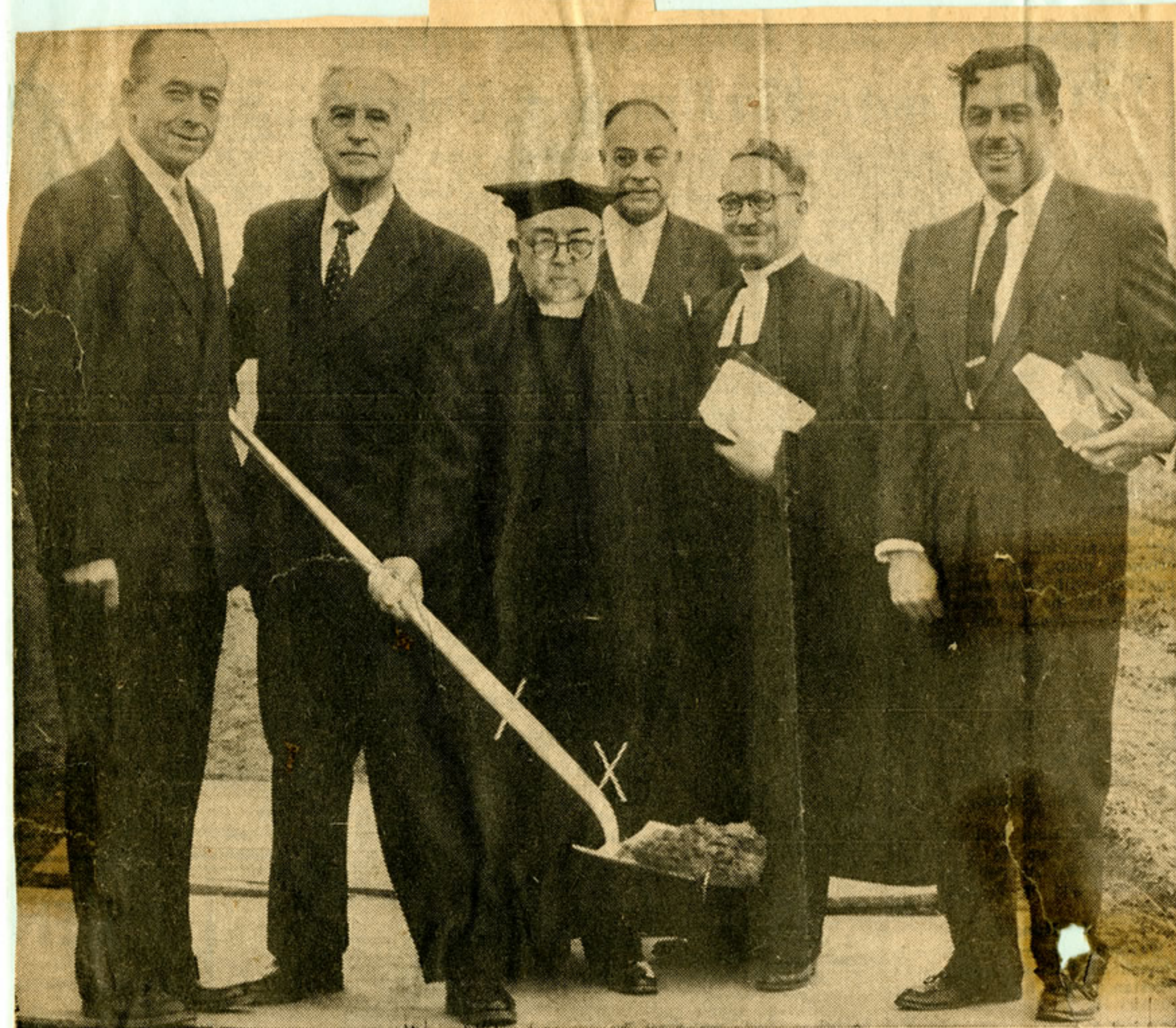
TURN SOD FOR NEW CHURCH — The congregation of the Aldershot Presbyterian Church, which is meeting temporarily in the auditorium of Glenview School, witnessed an auspicious occasion on Sunday following the morning service, when ground was broken for the new church building on LaSalle Park Road. Pictured at the occasion are, from the left, J. Frank Duff, clerk of session; W. J. Moffat of St. Paul's Presbyterian Church, Hamilton, convener of the extension committee of the Ham-
