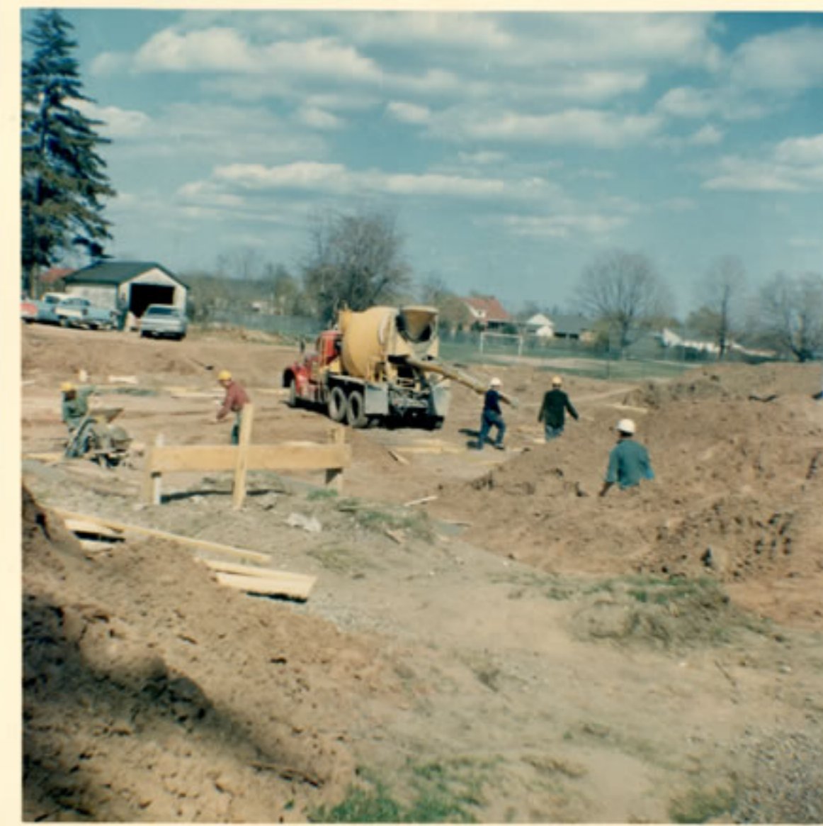
Pouring cement for new church -
