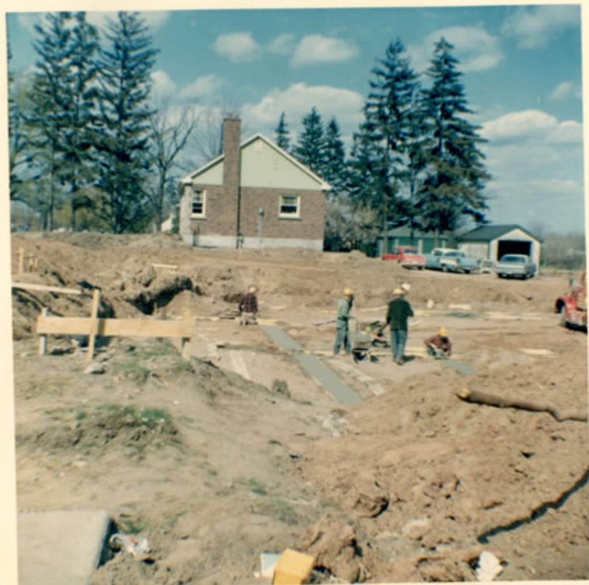
Excavation for new St. Matthew's Church -
