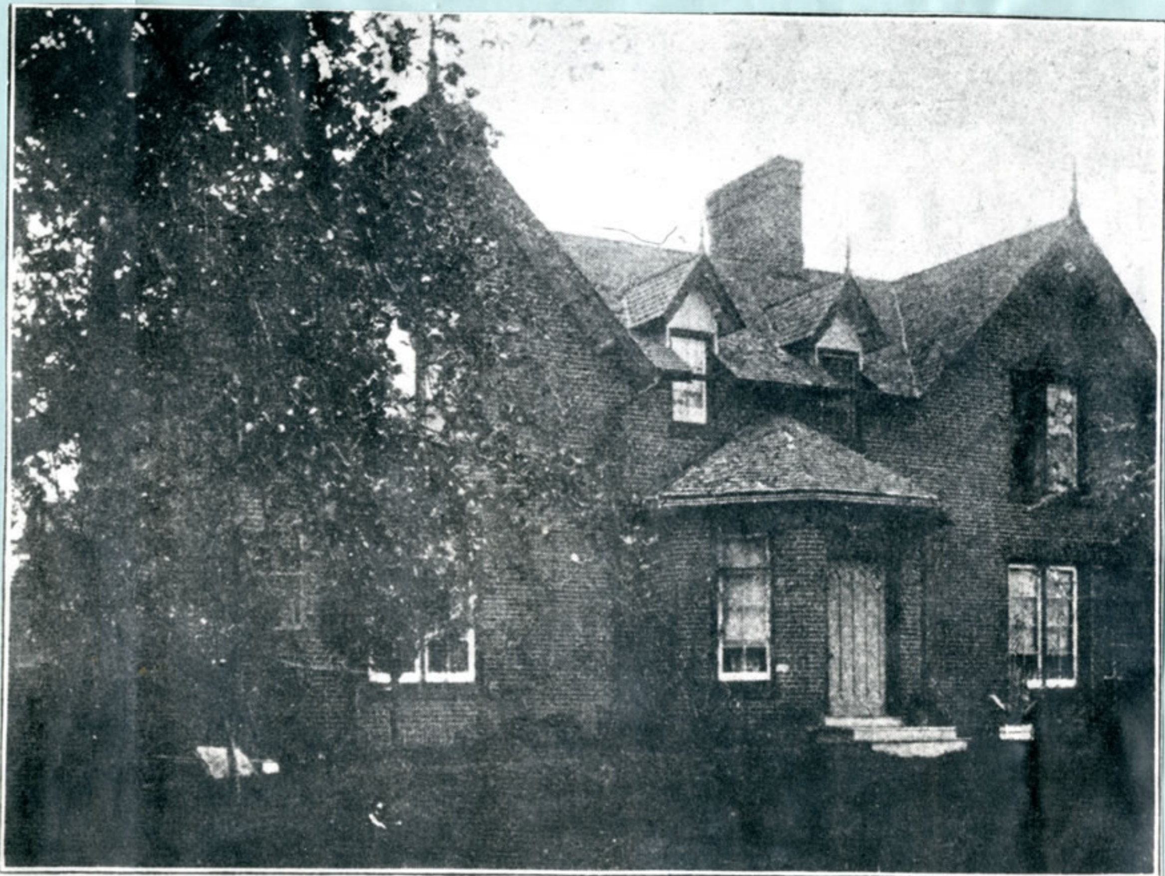
"HERBERTON HOUSE," RESIDENCE OF REID BROS., ALDERSHOT.
