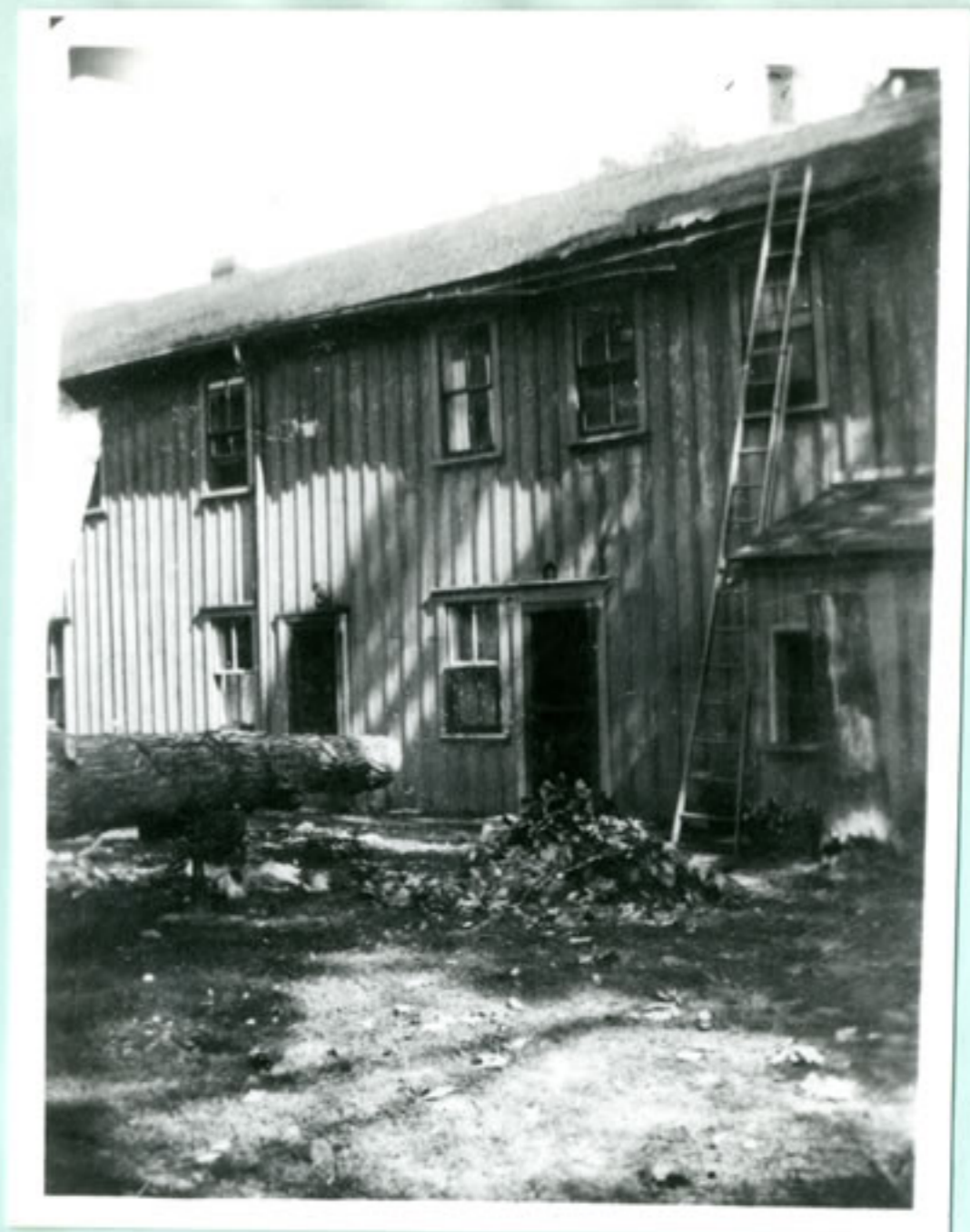
"Oaklands" damaged when huge oak tree fell upon it.
