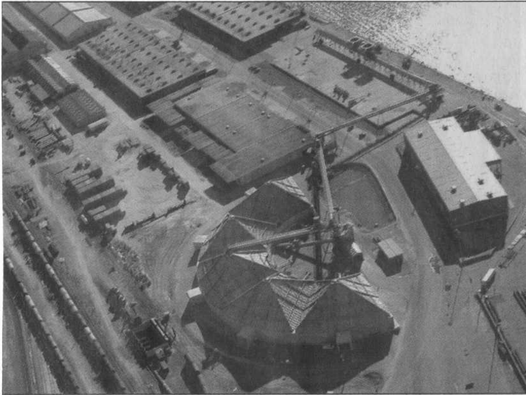
Aerial view of the Wilmington facility, designed and built by EMS-TECH.
