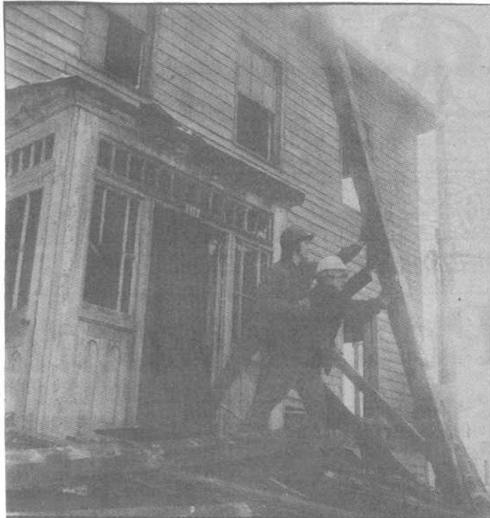
A demolition crew tears down the building.
