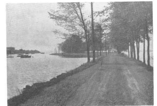
PROTECTED BAY AT VICTORIA PARK, BELLEVILLE
