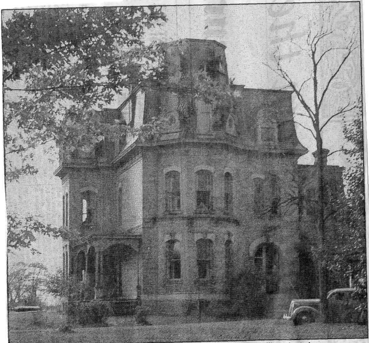
The former Albert College girls' residence when it was still a private home.
