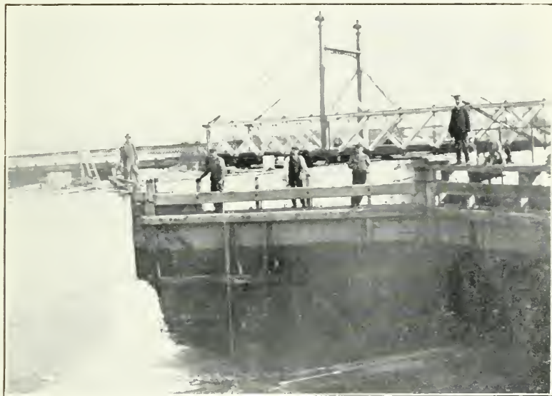
Lock 24, at Thorold, on the Eighteen-Seveny Canal, Dynamited by Fenians April 21st, 1900, showing headgates under repairs. United States soldiers' remains were discovered adjacent to this in the canal construction, re-interred, and monument erected.
