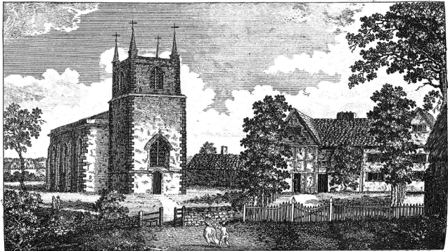
Abbeys Church & Rectory House
