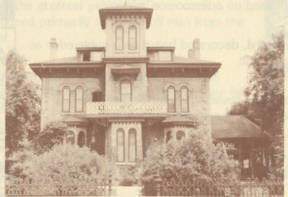
The Tisdale House, built in 1866-67 is one of the best examples of the Italianate house styles in Ontario and is the oldest and finest Italianate "villa" in Brantford. T.G. Tisdale, was the owner of the Brantford Stove Works and also one time councillor for the town of Brantford. 20-22 Nelson Street.
