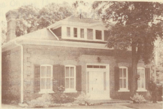
This building has a high hipped shingled roof with a dormer centred in the middle. One of the highlights of this house is the front entrance. It has recessed sidelights and a decorated transom with eye brown window. 89 Charlotte Street.
