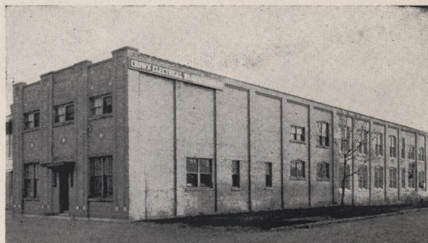
Crown Electrical Manufacturing Ltd.
