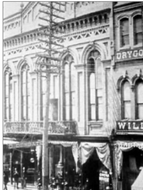
Street view of the Ker's Music Hall which later became the Stratford Opera House 2
