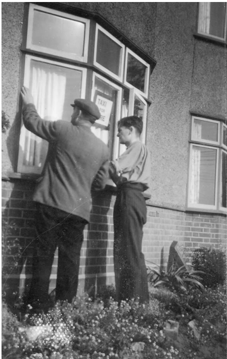
Repairing windows broken by bomb blasts
