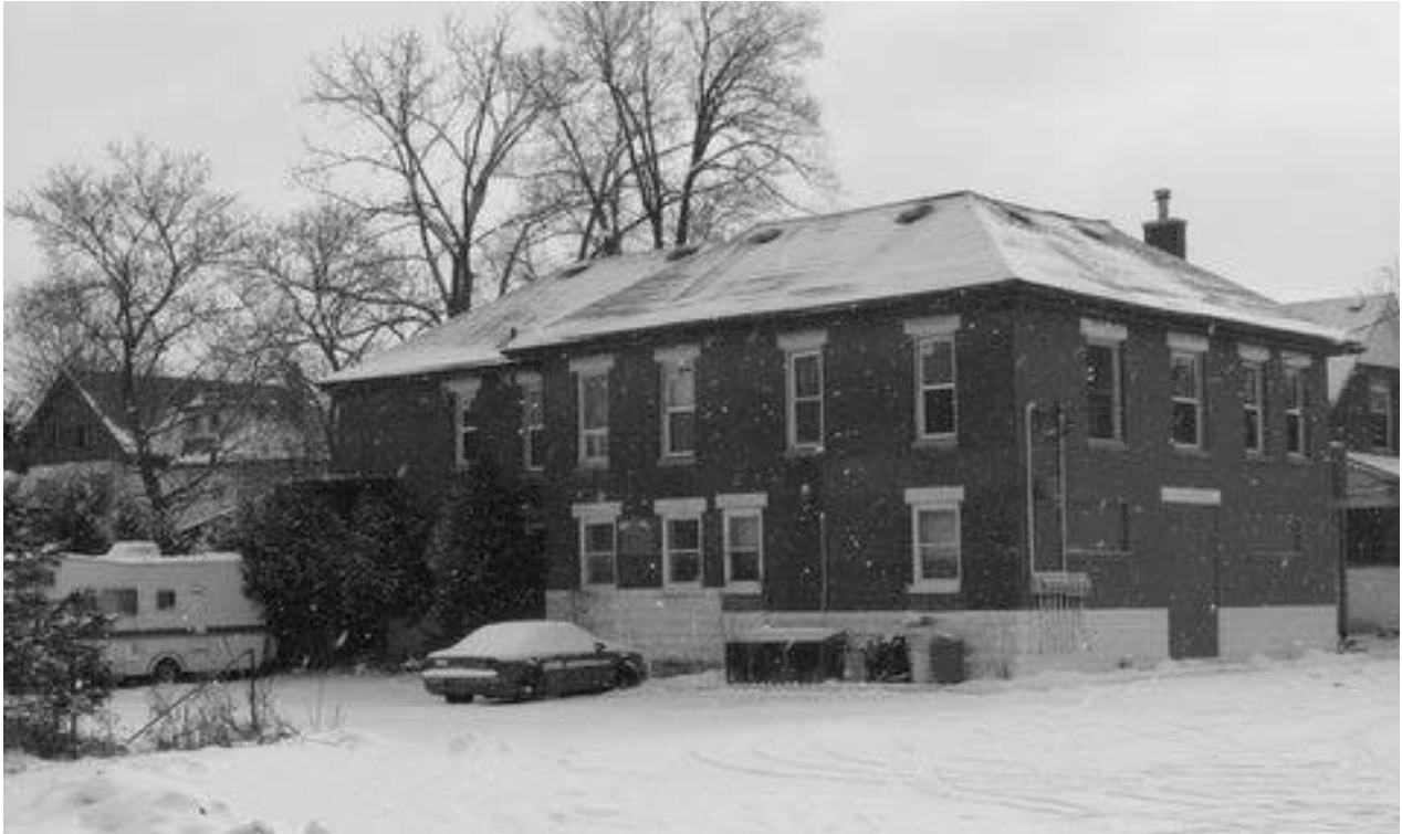
The Western Hotel in 2011. It is now an apartment building. The door in the centre of the right side, formerly the main entrance, is now filled in. It faces St. Catharine's street.
