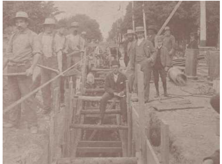
Picture above: City workmen on a sewer job on Colborne Street.
