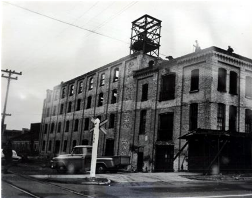
Dominion Radiator, Market Street
