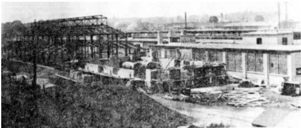
August 2nd, 1918 - Steel being erected on south side of building. Possibly intended as foundry. Never completed and eventually demolished
