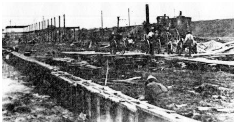
June 4th, 1918 - Steel being erected
