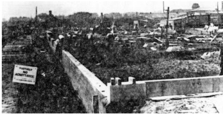
May 31st, 1918 - Foundation completed.
