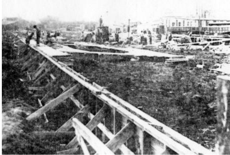
May 28th, 1918 - Foundations being prepared. Note steam powered cement mixer.
