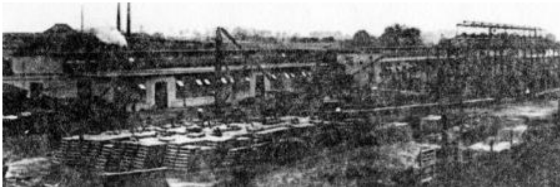
August 9th, 1918 - Note shell casings
