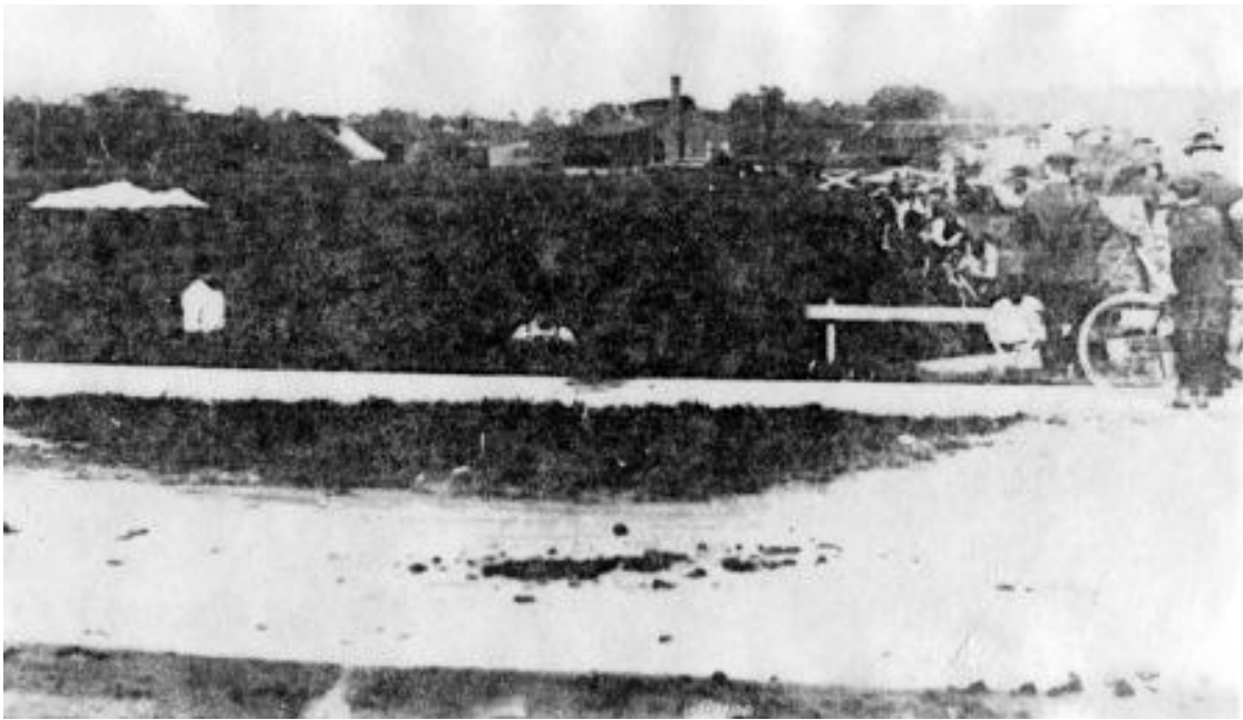
May 21st, 1918 - Construction commences. Railway runs along the embankment on the left and Murray Street is in the foreground.
