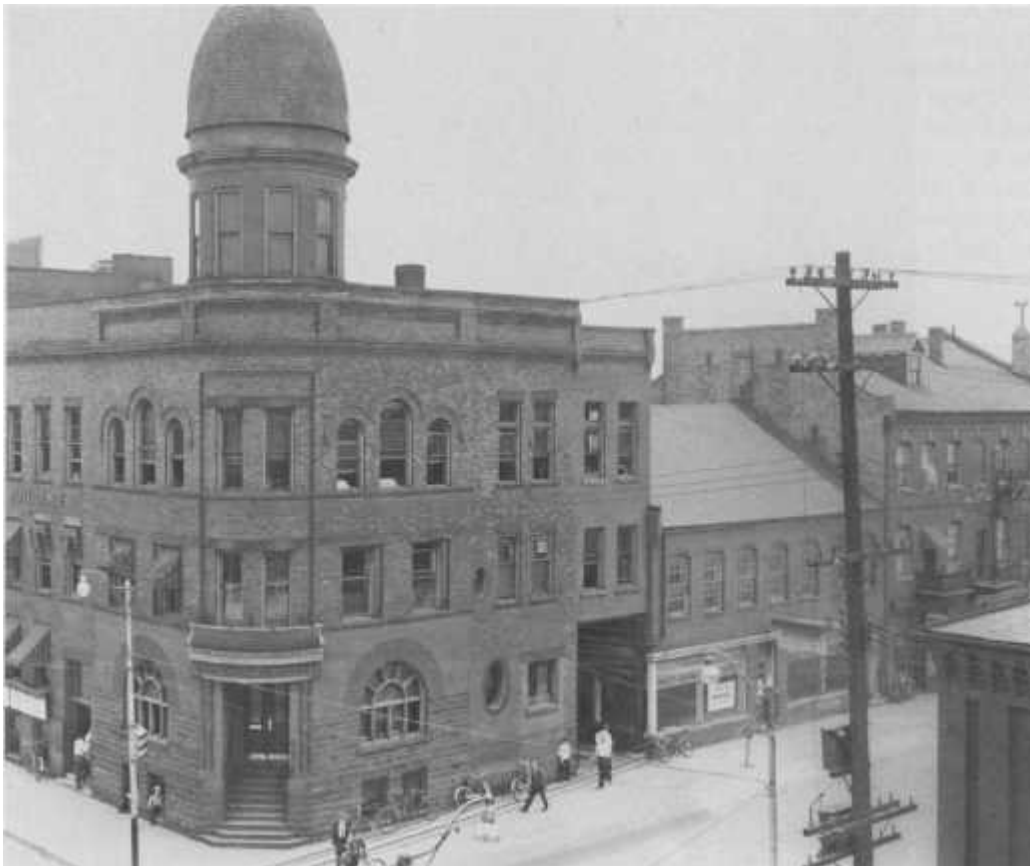
The Expositor before cupola was removed, and front doors re-sited.
