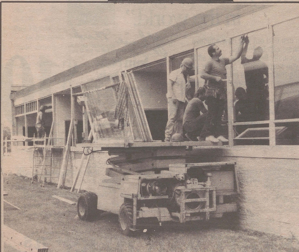
CONSTRUCTION workers make Van Lare Hall more energy efficient with new windows
