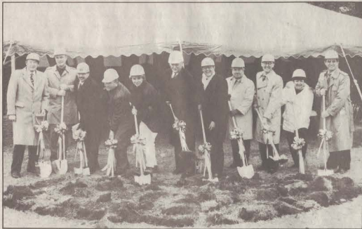
Ground breaking for "The Center" occurred in December. Approximately 200 people attended the ceremonies, including state politicians and local dignitaries.
