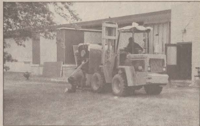
In 1990, the original boiler, installed in 1958, was replaced.
