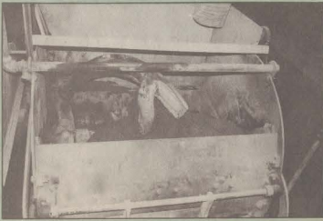
Aggregates and cement are mixed with water.
