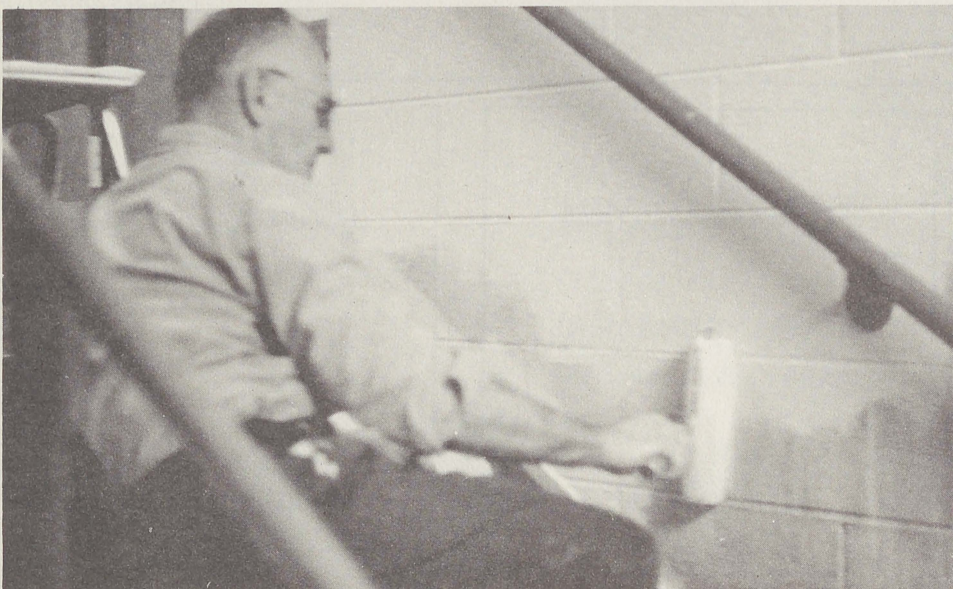
It takes alot of paint to cover the damage.
