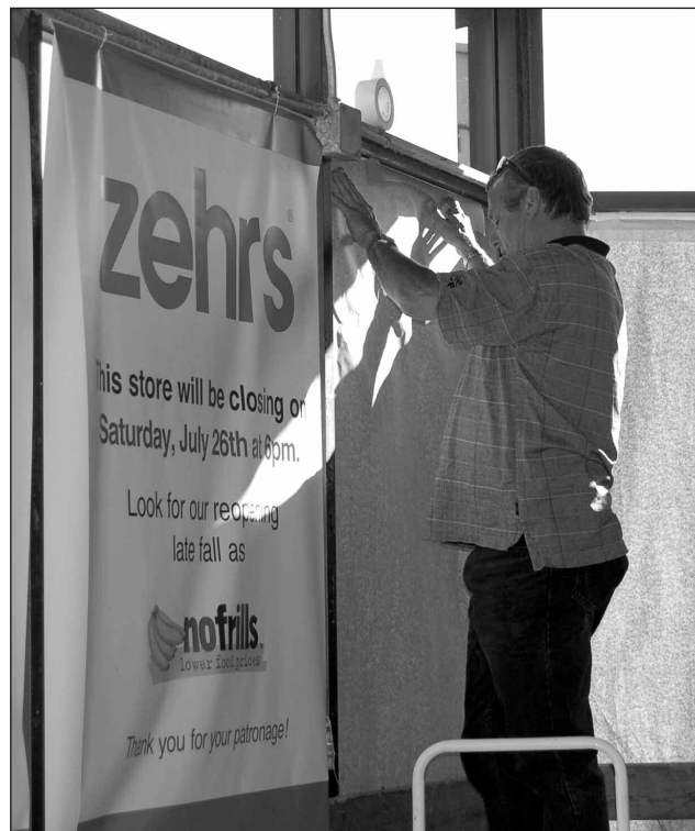
A member of the construction crew that will spend approximately two months converting Zehrs to No Frills puts brown paper over the front windows.
