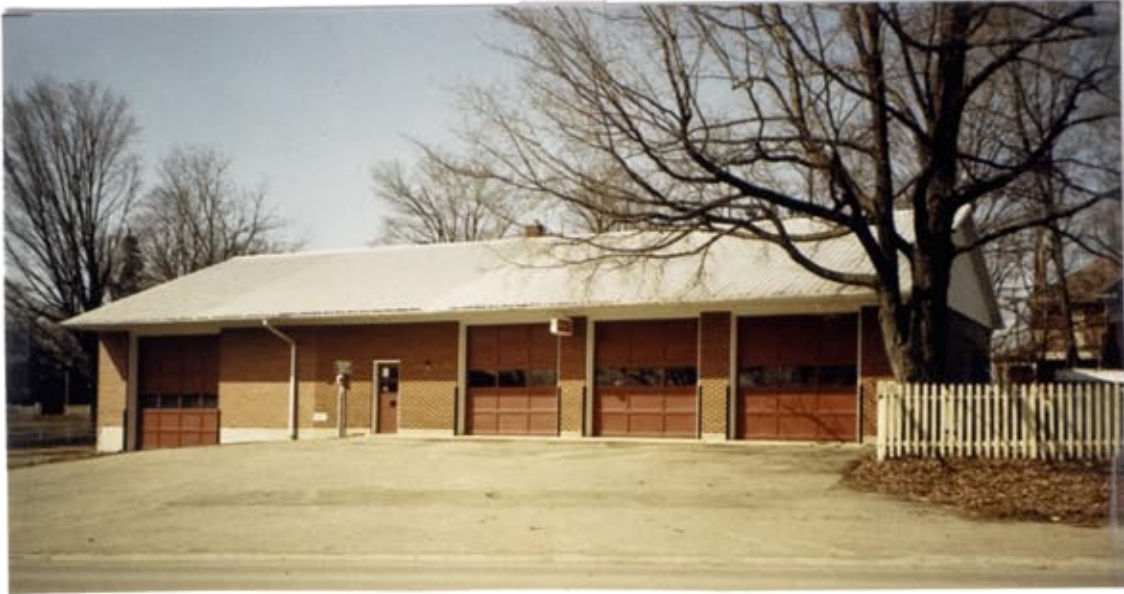
The new Fire Hall at Scotland.
