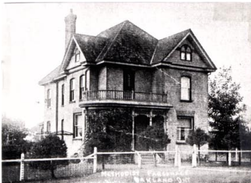
Circa 1900 - Oakland Methodist parsonage built in 1898 as shown on the glass window at the front door.
