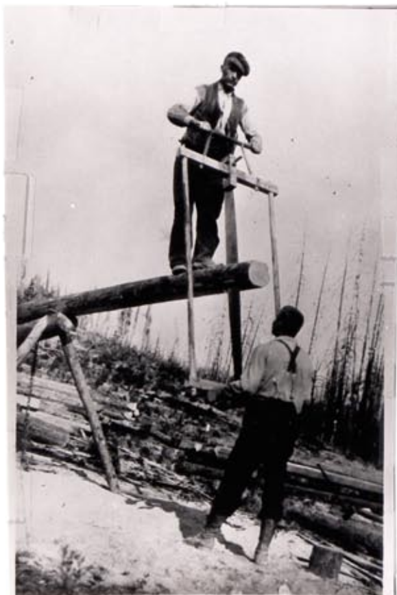
Two men cutting lumber with a gate saw (whipsaw). The sawyer at the bottom got a shower of sawdust as the log was cut on the down stroke.
