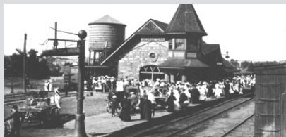
Grand Trunk Station 1908
