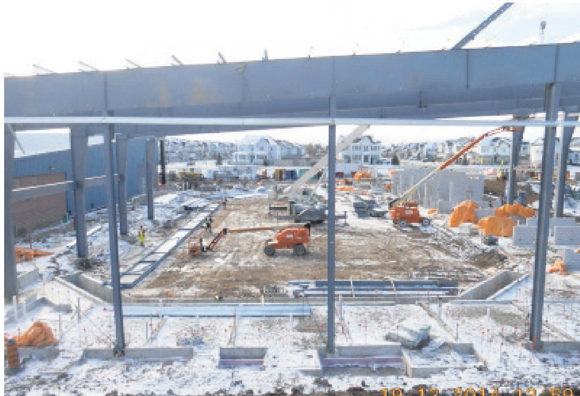
Steel is being erected on the new arena addition at the Acton Arena & Community Centre.
