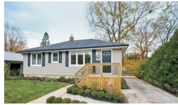
RENOVATED TOP TO BOTTOM - INSIDE & OUT $249,000 www.latamandlatam.com 13-466 X2763744
