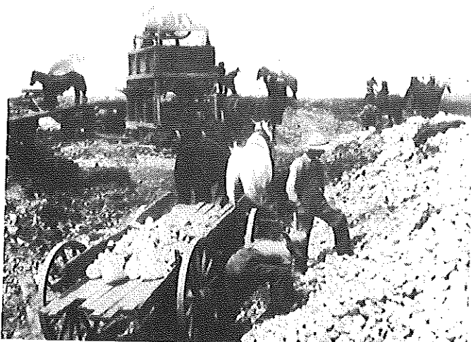
In William Kennedy's gravel pit, Joe Ritchie's Sawyer-Massey operating the crusher. William and George McCulloch loading stones to be crushed.
