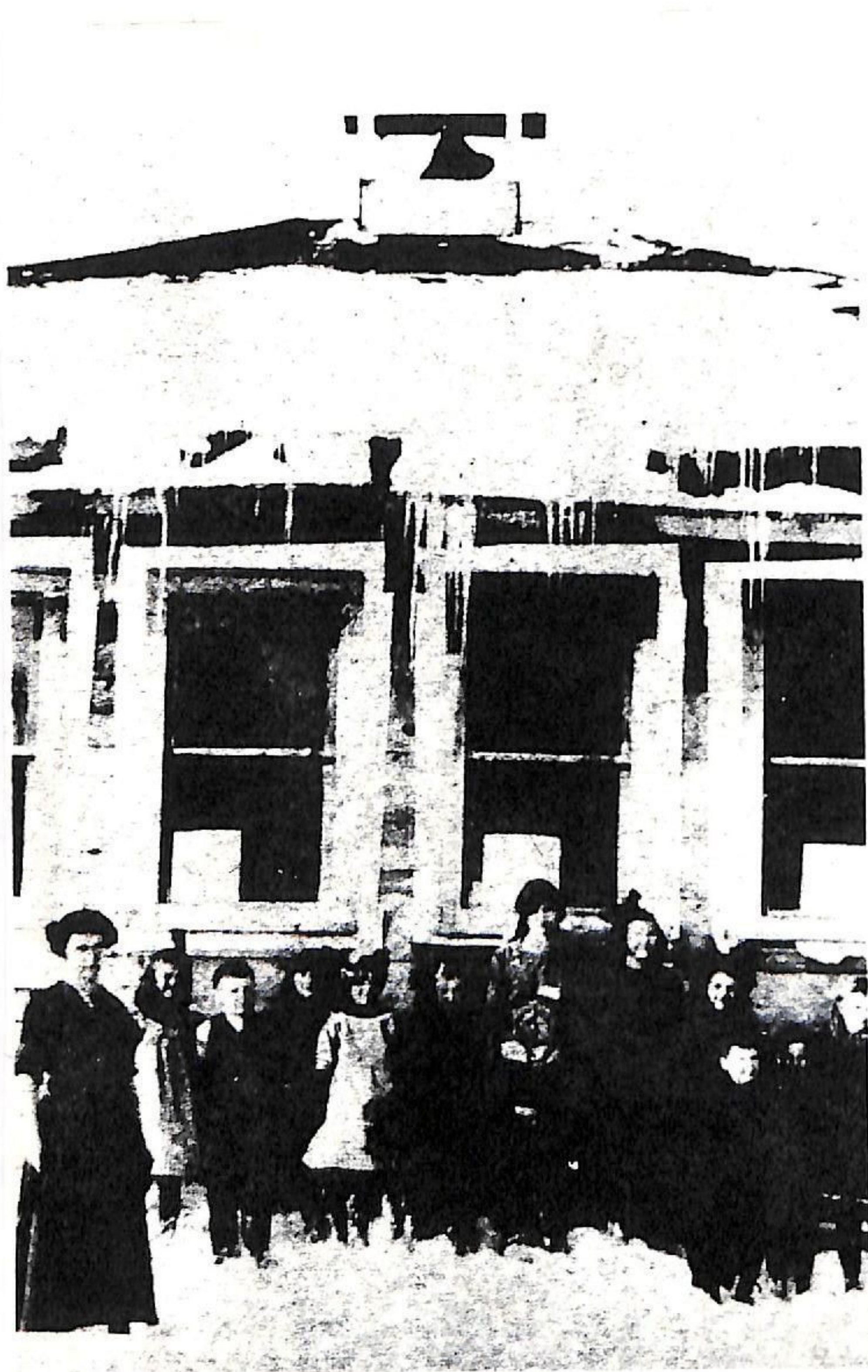
Kelso Settlement, Cochrane District, Ontario
